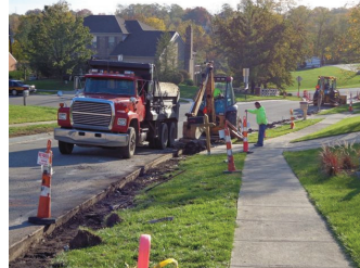
Crew working on curb replacement Abbey Court - part of the Annual Street Rehabilitation Contract.
